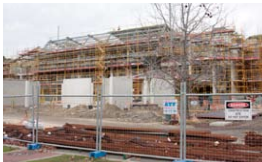
Yes, the building is actually taking shape! We look forward to moving in and seeing you there. (Photo: R.Barrett)
