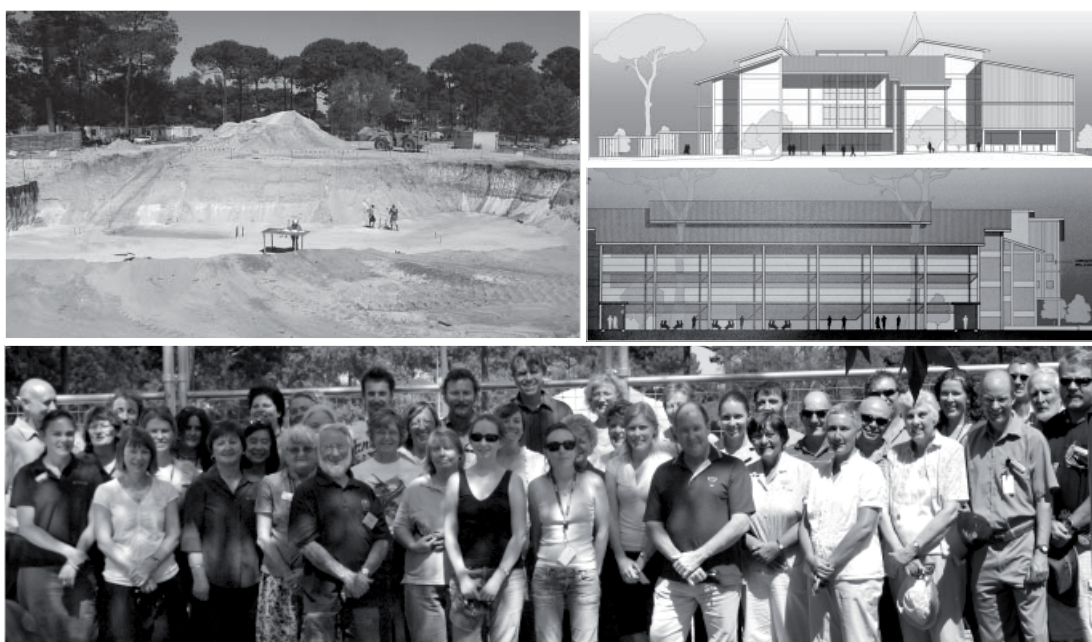
Fig. 1. (From top left, anticlockwise). a, Biodiversity Science Centre construction work, 25 th Jan 2008; b, staff visit that day; c, Biodiversity Science Centre north elevation and d, west elevation. Ph. K. Thiele
